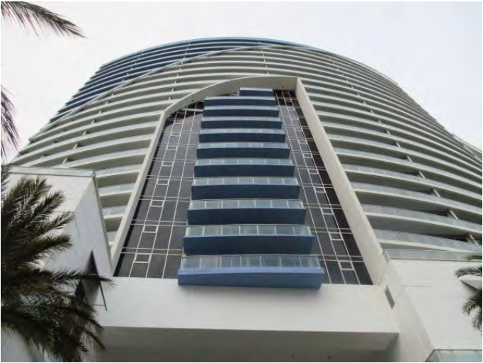
GENERAL VIEW OF BUILDING EXTERIOR FINISHES
