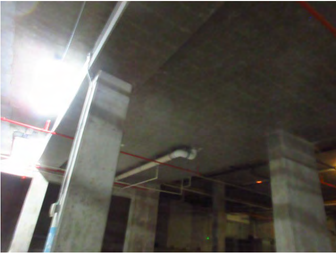
GENERAL VIEW OF SUPERSTRUCTURE
