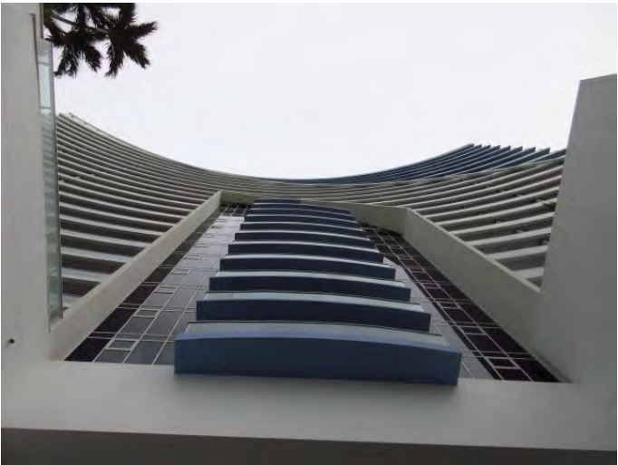
VIEW OF BUILDING EXTERIOR FINISHES
