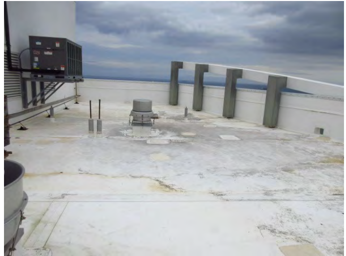
VIEW OF ROOF COVERING
