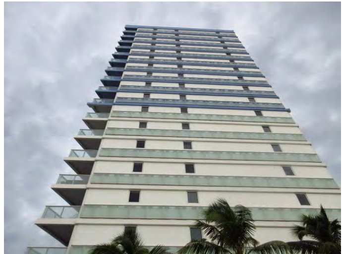
VIEW OF BUILDING EXTERIOR FINISHES
