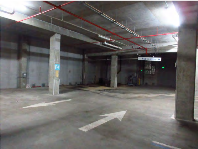
GENERAL VIEW OF PARKING GARAGE
