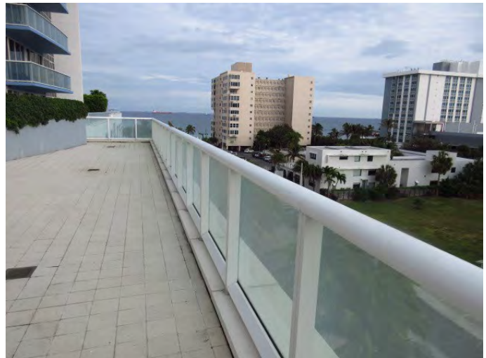
GENERAL VIEW OF BALCONY RAILING
