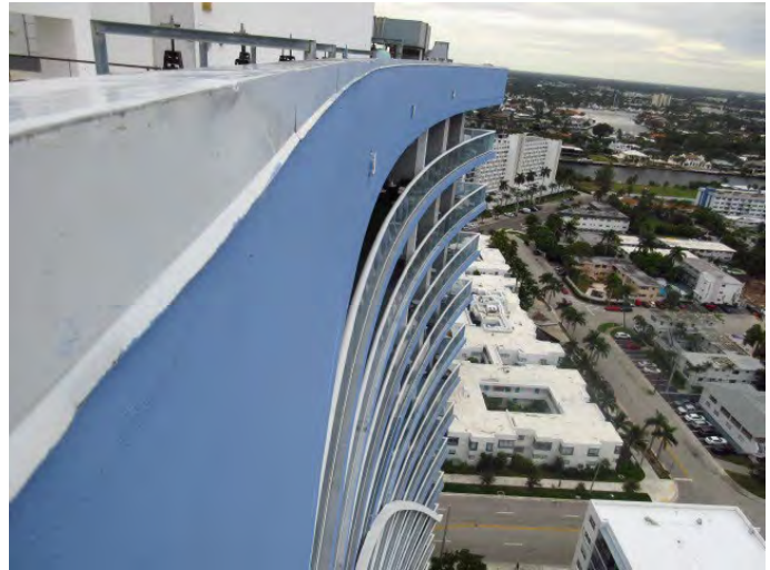
VIEW OF BUILDING EXTERIOR FINISHES
