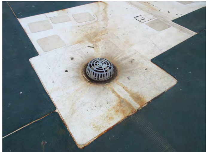
VIEW OF ROOF DRAIN
